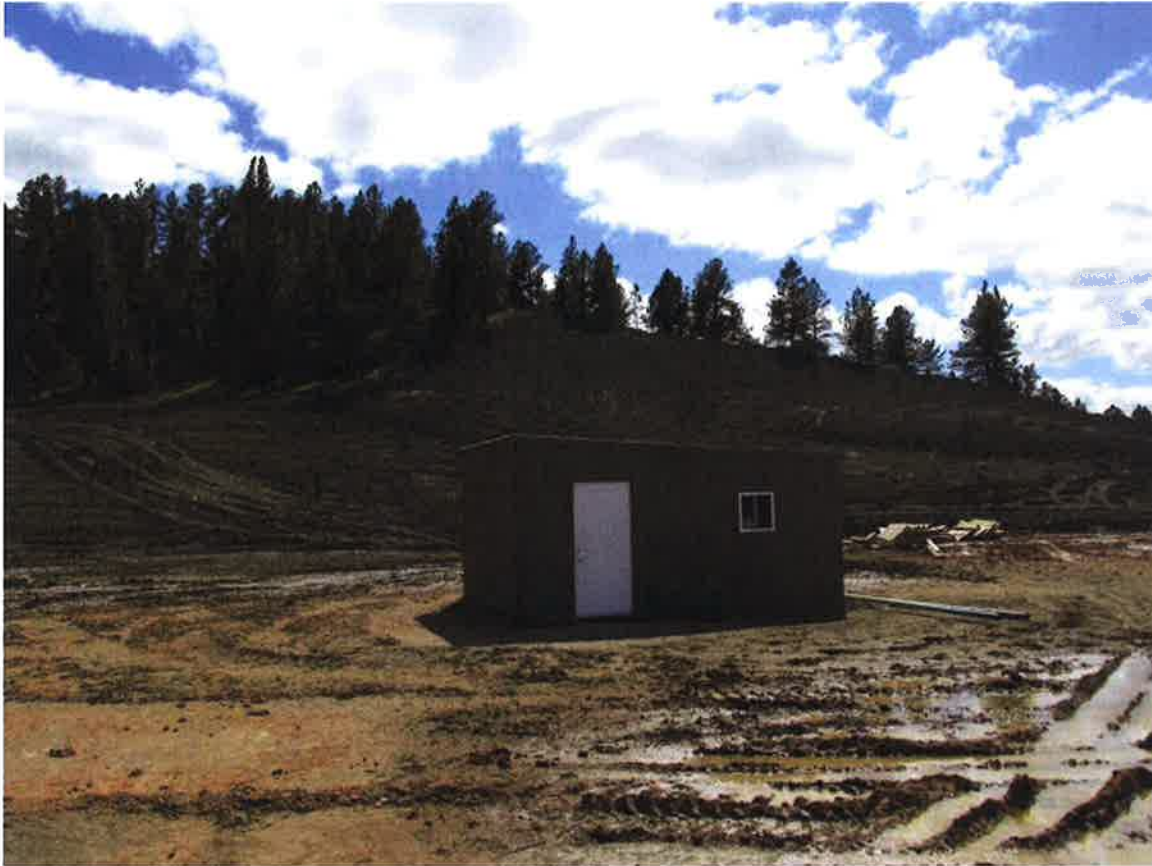
Photo of existing well site showing steep cut behind the building toward the top of the slope and introduced road material in the foreground.
