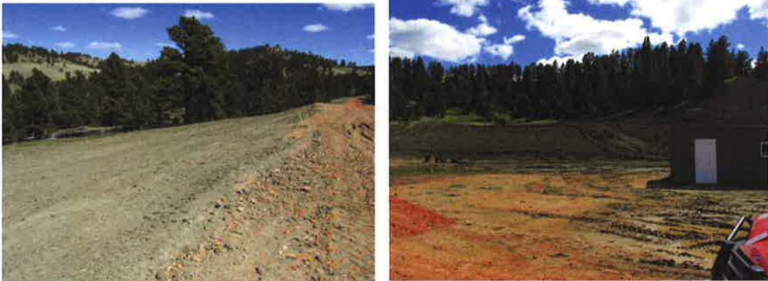
Native soil is the darker material. Red soil has been brought in as road material.
